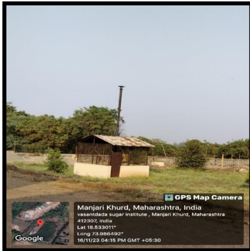
Incinerator installed for solid waste
